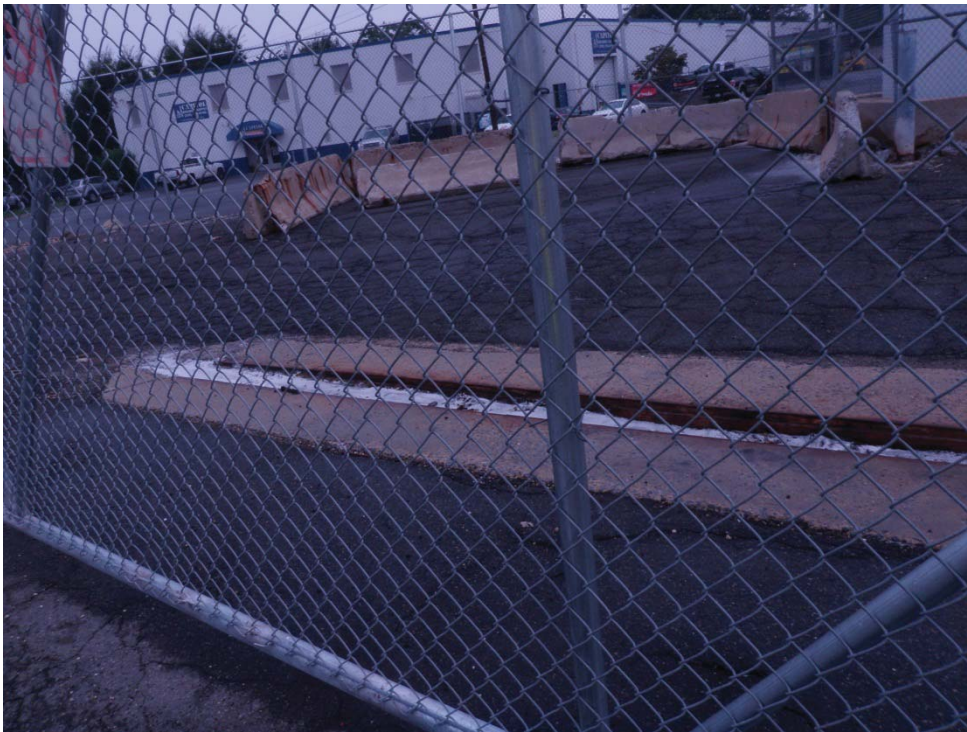
Photo #6: Sump in southwestern portion of subject site
