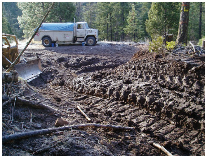
Figure 43—Severe rutting from harvesting on top of moist soil.
