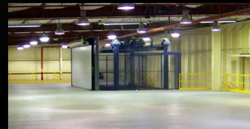
Boat Mold Lift – F Series Mechanical VRC Retrofitted design doubled storage space for fiberglass mold dollies in lamination production area. 5,000 lbs. lifting capacity.
